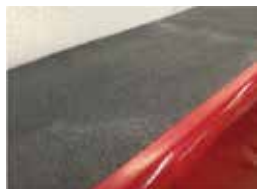
Anti-slip runway traction surface
